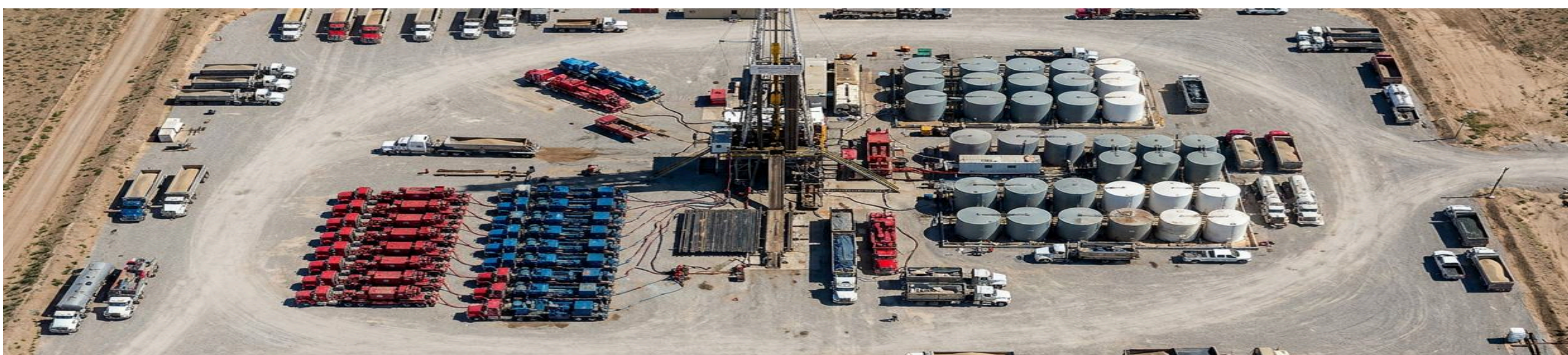
Overhead imagery from a multi-well shale pad — Permian Basin, Texas. Structural classification applied across full pad footprint.
